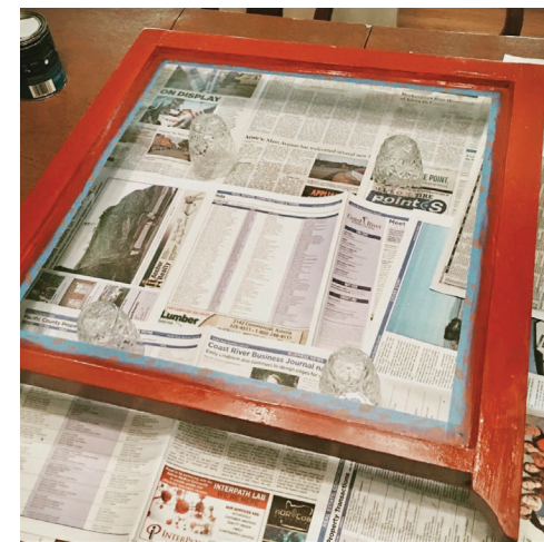
The top window of an 1894 double hung sash window in the pantry of the Forsstrom House.
