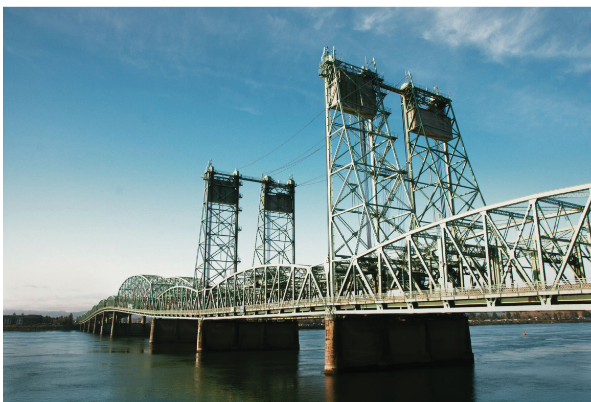
ABOVE: The Interstate Bridge, which connects Portland and Vancouver. BELOW: The Dalles Bridge crosses near the Indian Shaker Church ruins.
