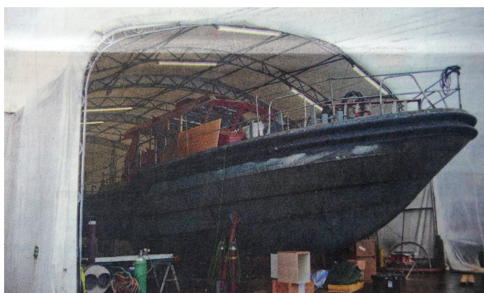
The Connor Foss, a new bar pilot launch vessel under construction at the Foss Maritime boatyard in Rainier, seen in 2012.
