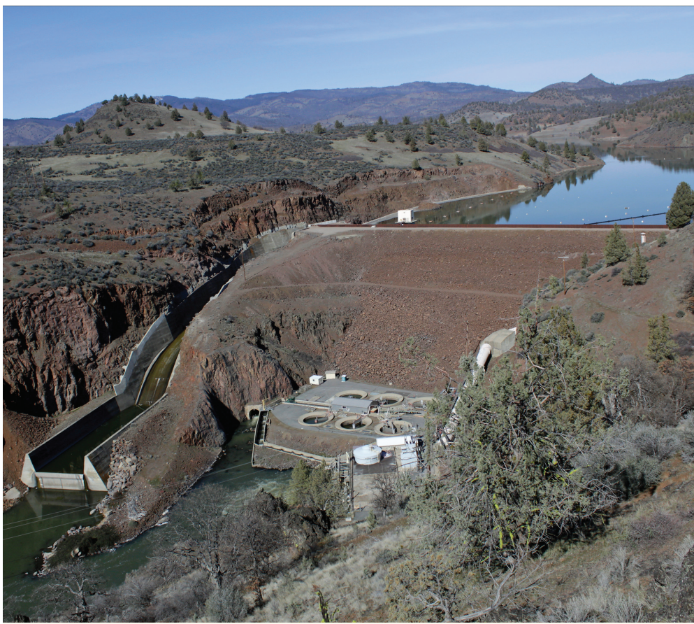
Gillian Flaccus/AP Photo The Iron Gate Dam, powerhouse and spillway on the lower Klamath River near Hornbrook.
