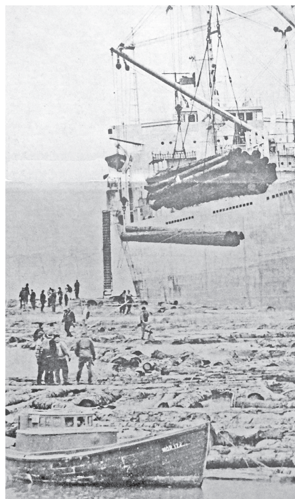
Work at the Port of Astoria in 1972.
