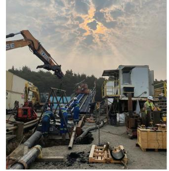
Oregon State University Crews drill tunnels for underground cables connecting the wave energy capturing devices and the power grid connection facility at Driftwood State Recreation Site.
