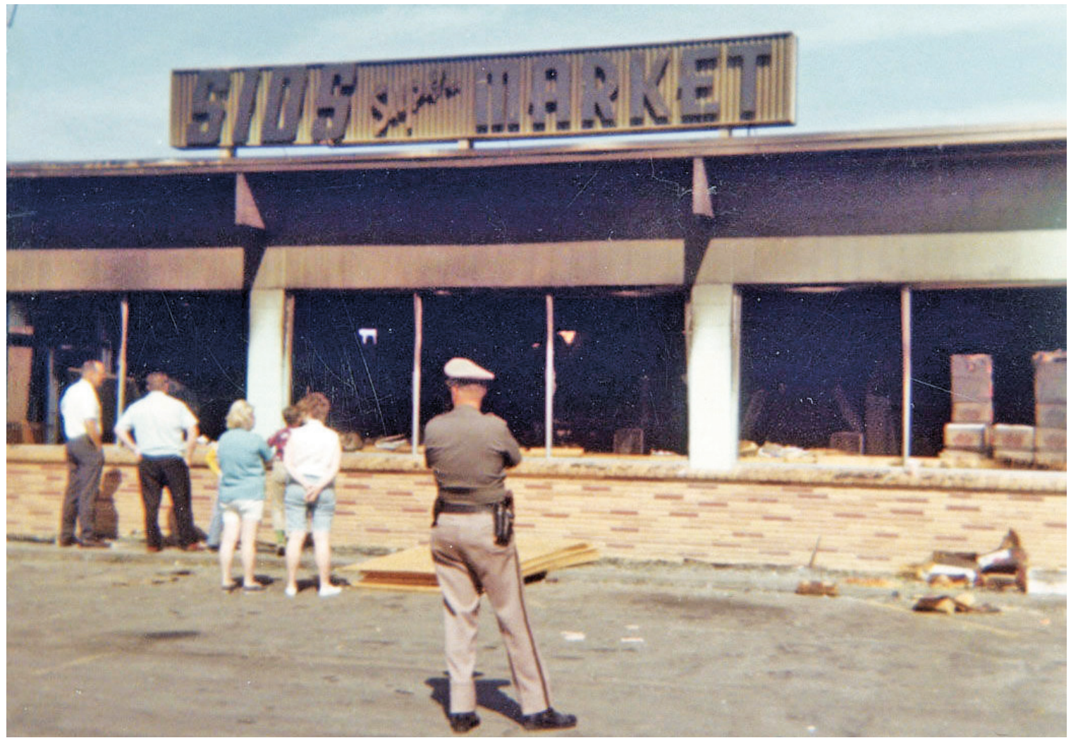
A photo of the burned Sid’s Market after the fire.
