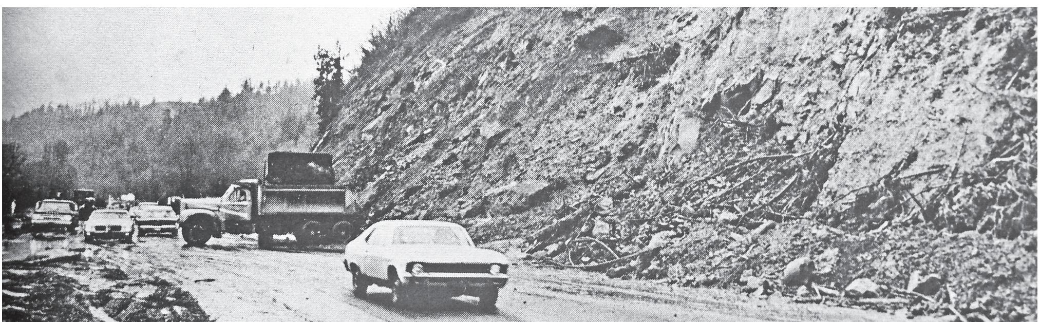
State highway officials worked to address an area prone to slides near Westport in 1971.
