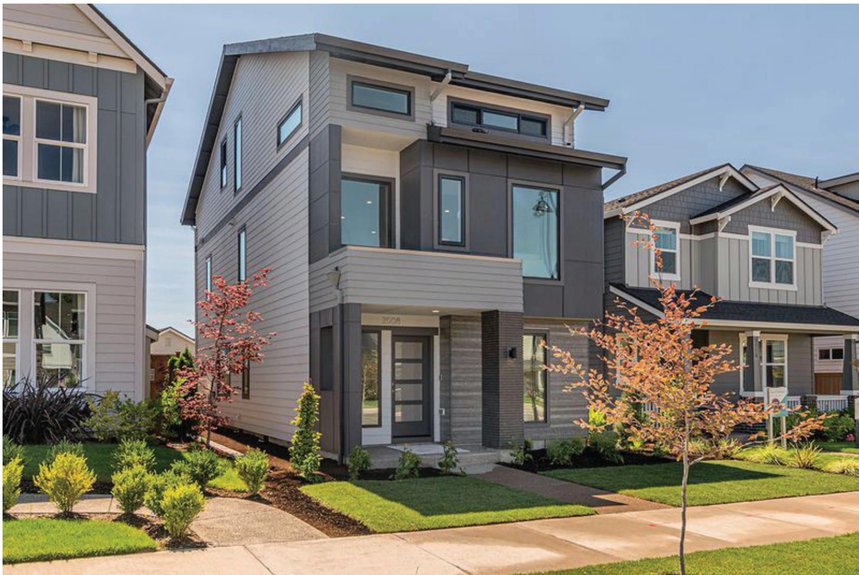
A solar-ready, all-electric house designed and constructed by Ichijo USA is seen in Hillsboro's Reed's Crossing.
