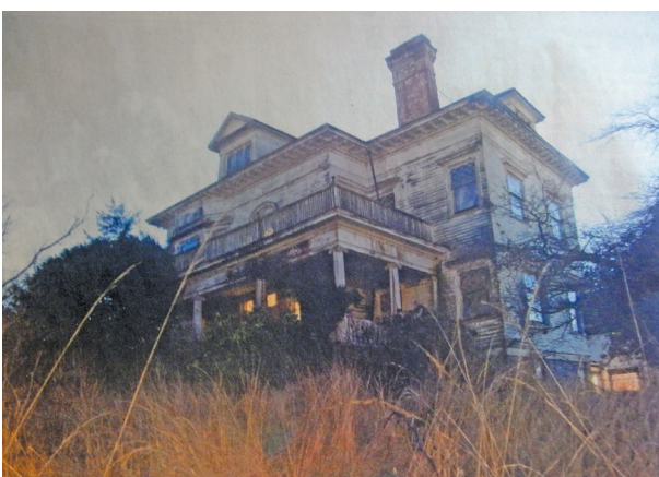
The abandoned Flavel home on the corner of 15th Street and Franklin Avenue in 2011.
