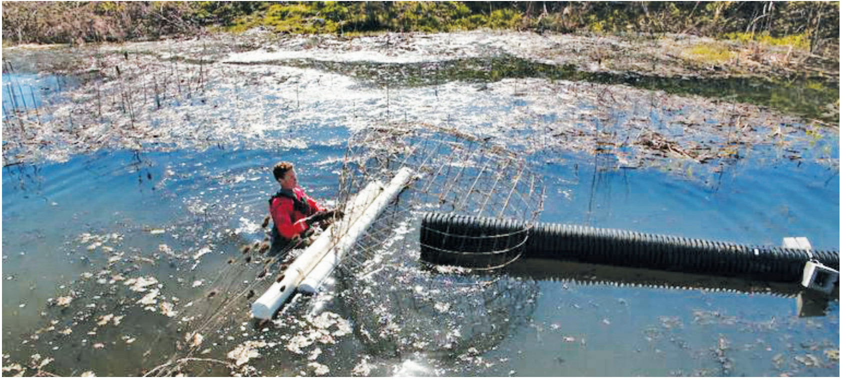
Jakob Shockey floats a pond leveler out into the middle of the beaver pond in Phoenix. The device acts like a bathtub overflow drain, preventing the pond from growing any bigger, no matter how high the beaver builds the dam.
