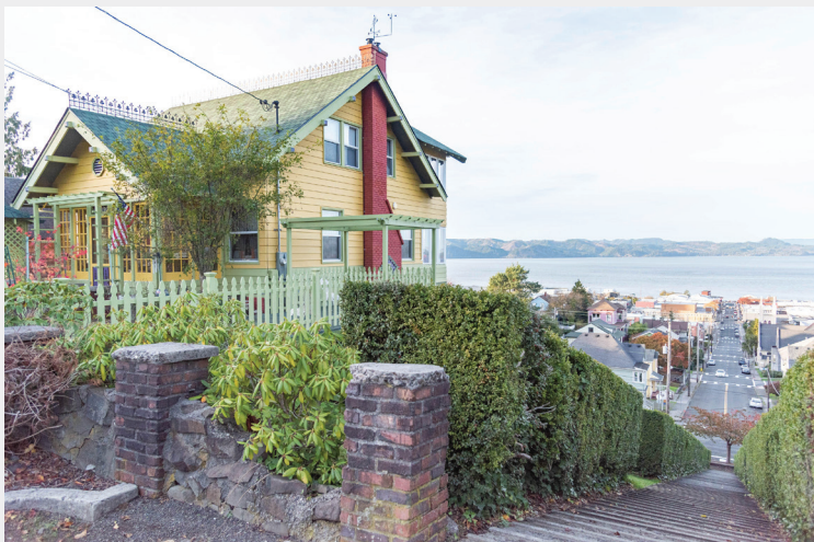
Billie O'Neel acknowledges she did work on her property without the necessary city approvals.
