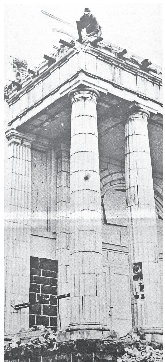
Crumbling columns at Clatsop Community College's Towler Hall seen in 1971.
