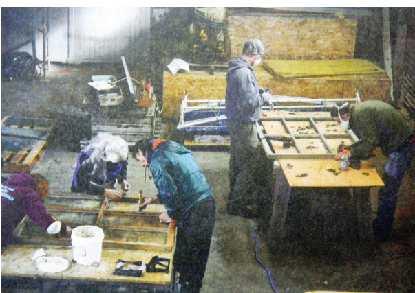
Students in Lucien Swerdloff's Clatsop Community College historic preservation class refurbish windows in the Astoria train depot in 2011.
