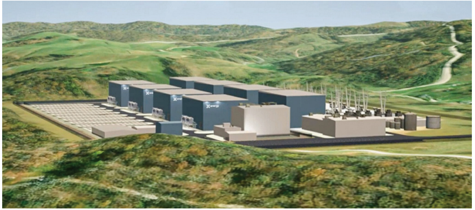
This rendering shows a proposed nuclear power plant by Maryland-based X-energy that would produce electricity from four helium gas-cooled reactors.
