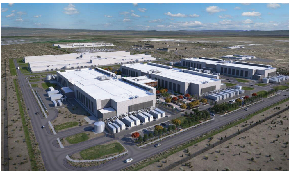
The Facebook data center in Prineville.
