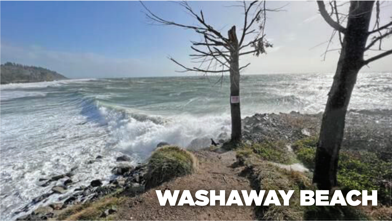
Jeff Clemens/Chinook Observer Powerful waves tear away at the shoreline at Washaway Beach in Pacific County, one of the fastest-eroding places on the West Coast.
