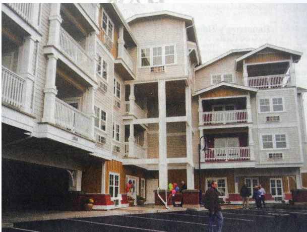
The 33-unit, four-story Astoria Gateway II affordable housing complex welcomed visitors to tour the new development in 2011.
