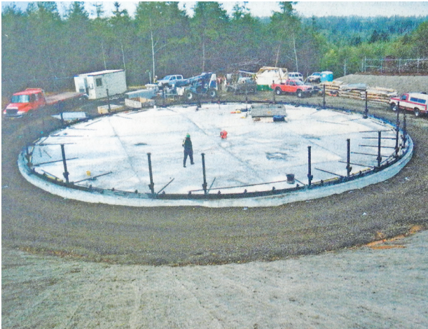
A 1 million gallon steel reservoir tank under construction east of Gearhart in 2011.
