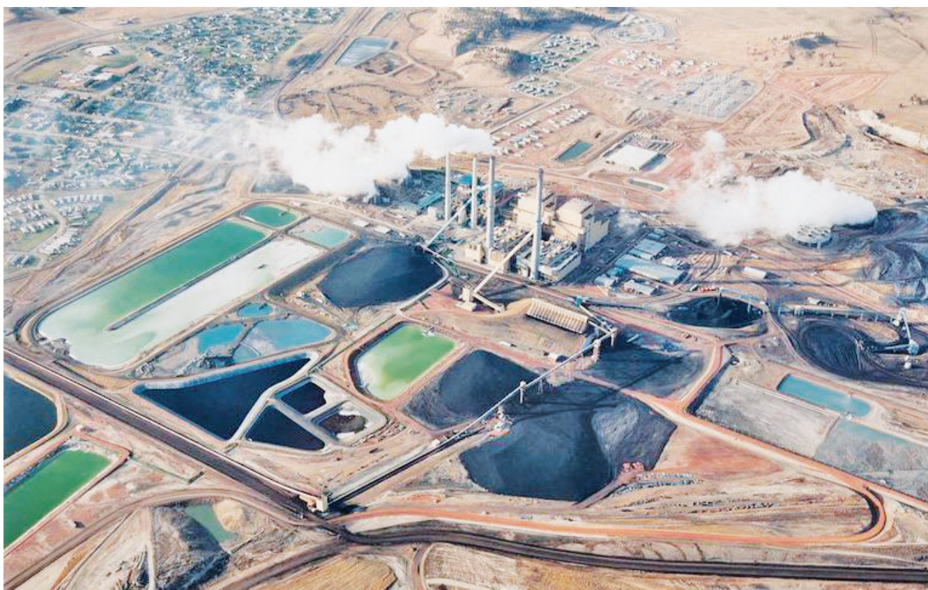
The Colstrip coal plant in Montana, which supplies electricity to customers in the Northwest and elsewhere.
