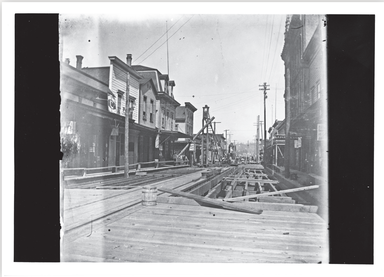
TOP: This photo circa 1896 shows the wooden pilings that made Astoria susceptible to fire. BOTTOM: The Astoria waterfront in 1880.
