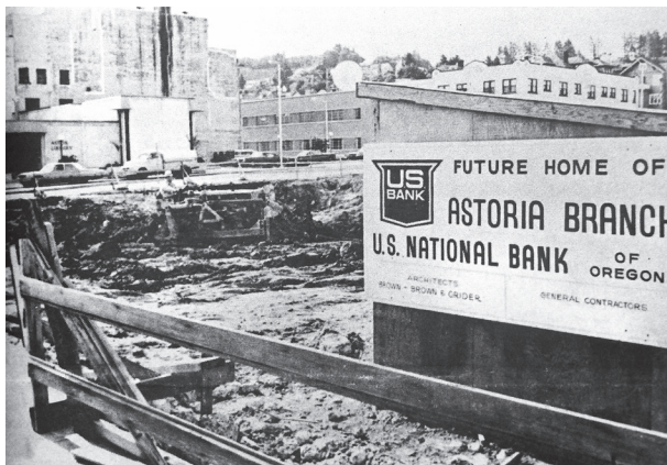
Construction of U.S. Bank in Astoria in 1971.
