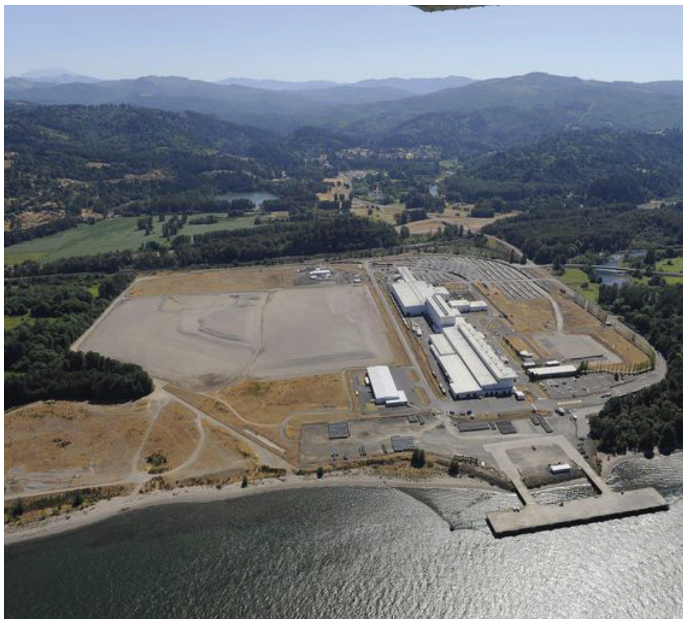
NW Innovation Works
