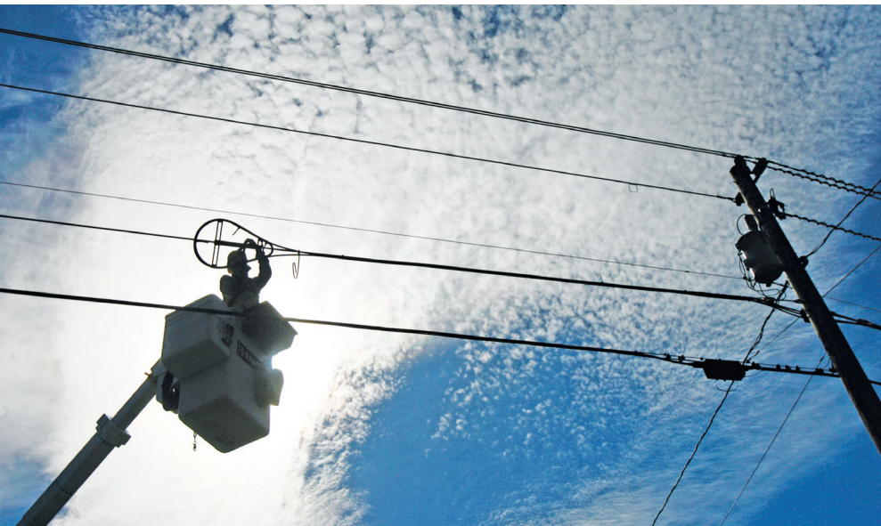
A.J. Bowen, of Schupp's Line Construction Inc., works on fiber-optic installation in Vermont in 2007.
