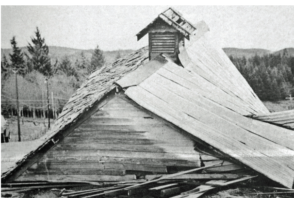
A building is damaged after a 1971 storm.
