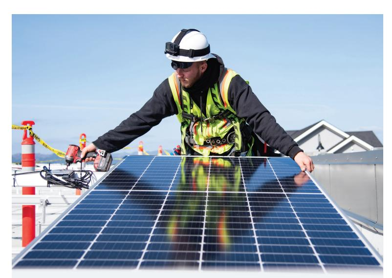
TOP: Garrett Lyle, from Elemental Energy, installs the first solar panel on the roof of the Astoria Co+op on Wednesday afternoon. The 51-kilowatt solar array is expected to generate about a third of the grocer's electricity. RIGHT: Co-op general manager Matt Stanley looks at the new solar panels. BELOW: Elemental Energy installs solar panels on the roof.
