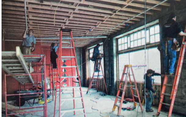
Workers with Seaside's Butler Construction work on framing along the wall of the Amazing Stories comic book shop in the Astor Hotel in preparation for installing sheetrock in 2011 after water damage.
