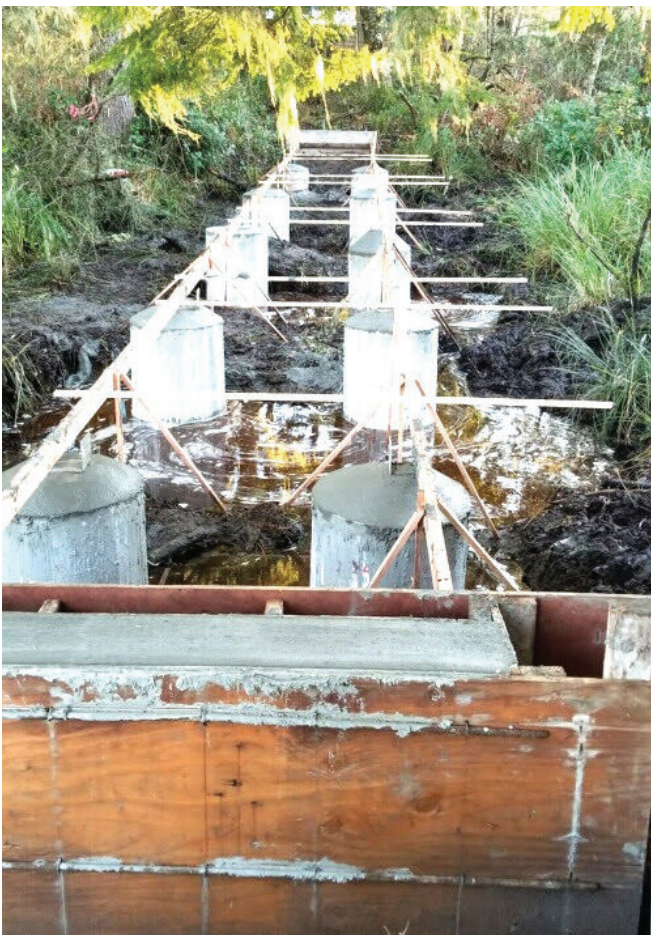
The concrete base to hold the bridge.
