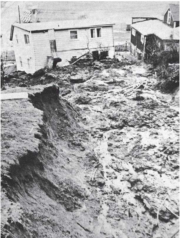
A mudslide sent David Kindred's home downhill in 1971.
