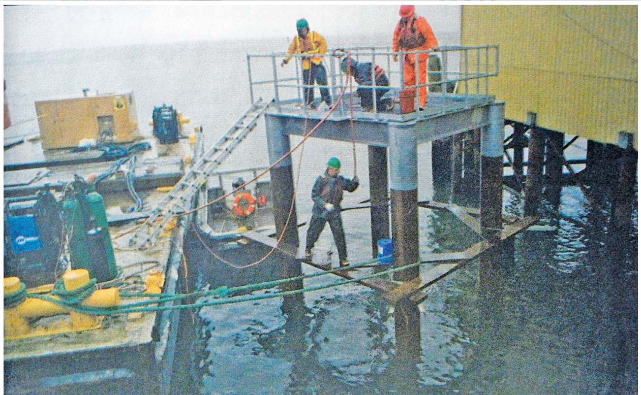
Work continued on a new Columbia River navigation aid in the water at the foot of Seventh Street in 2011 after the previous one was demolished in the No. 10 Sixth St. building fire.
