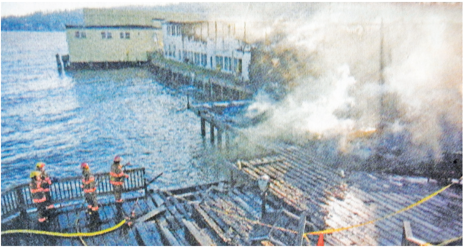
Firefighters monitor hot spots and spray water onto the Columbia River side of the No. 10 Sixth St. building after fire engulfed and burned it in 2010.
