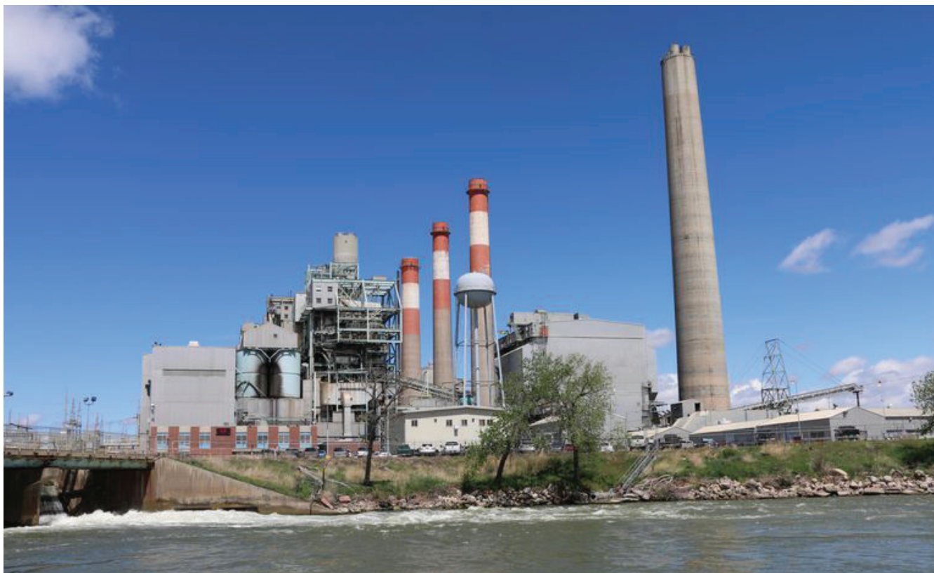
PacifiCorp's Dave Johnston coal-fired power plant in Wyoming is scheduled for retirement in 2027.
