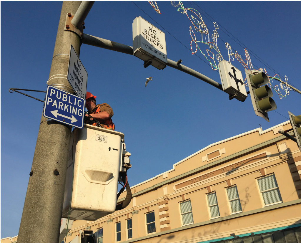
Crews at work on Holladay and Broadway in Seaside in fall 2018.
