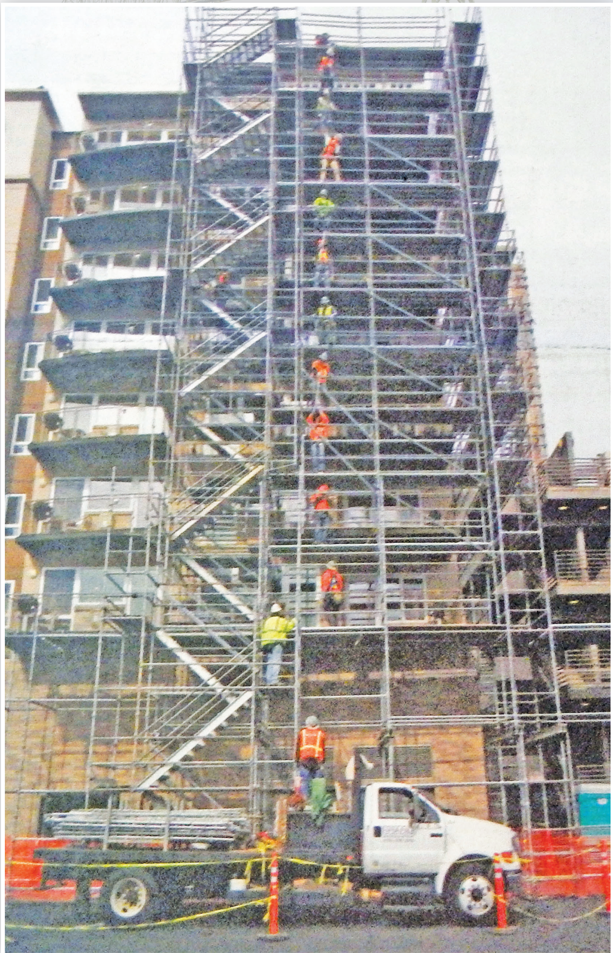
Workers form a vertical assembly line while hauling up pieces of scaffolding from a truck below to the top of the WorldMark Seaside in 2010.
