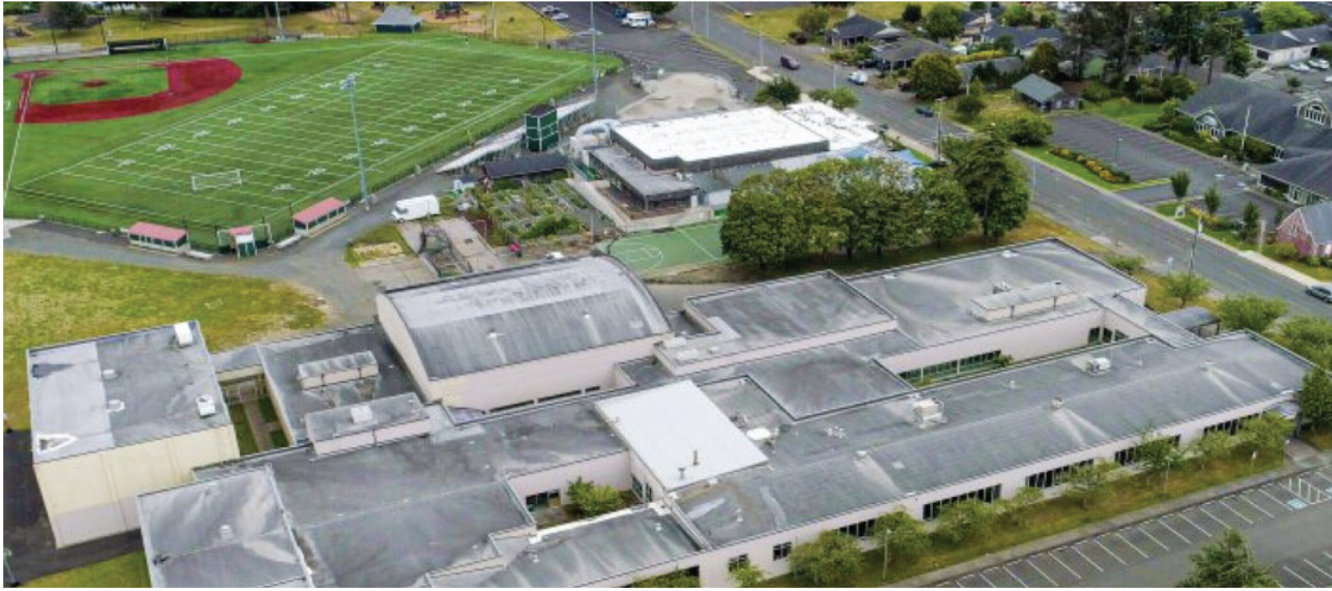
An aerial view of Broadway Middle School. Sunset Empire Park and Recreation District is located at top right-center.
