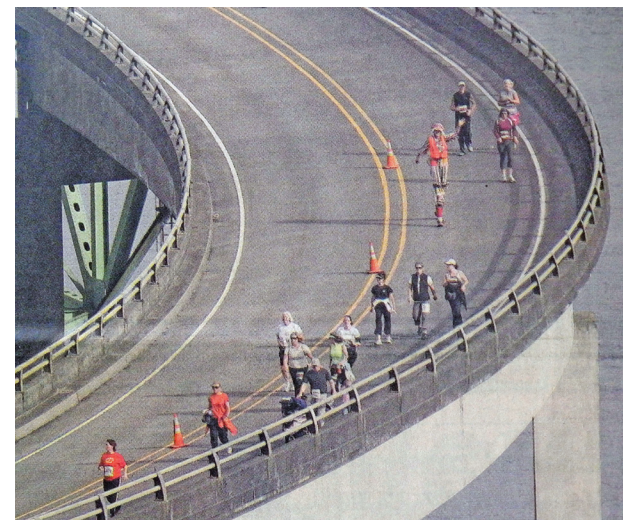
Runners, walkers and even a person on stilts, top right, near the finish line of the Great Columbia Crossing in 2010.
