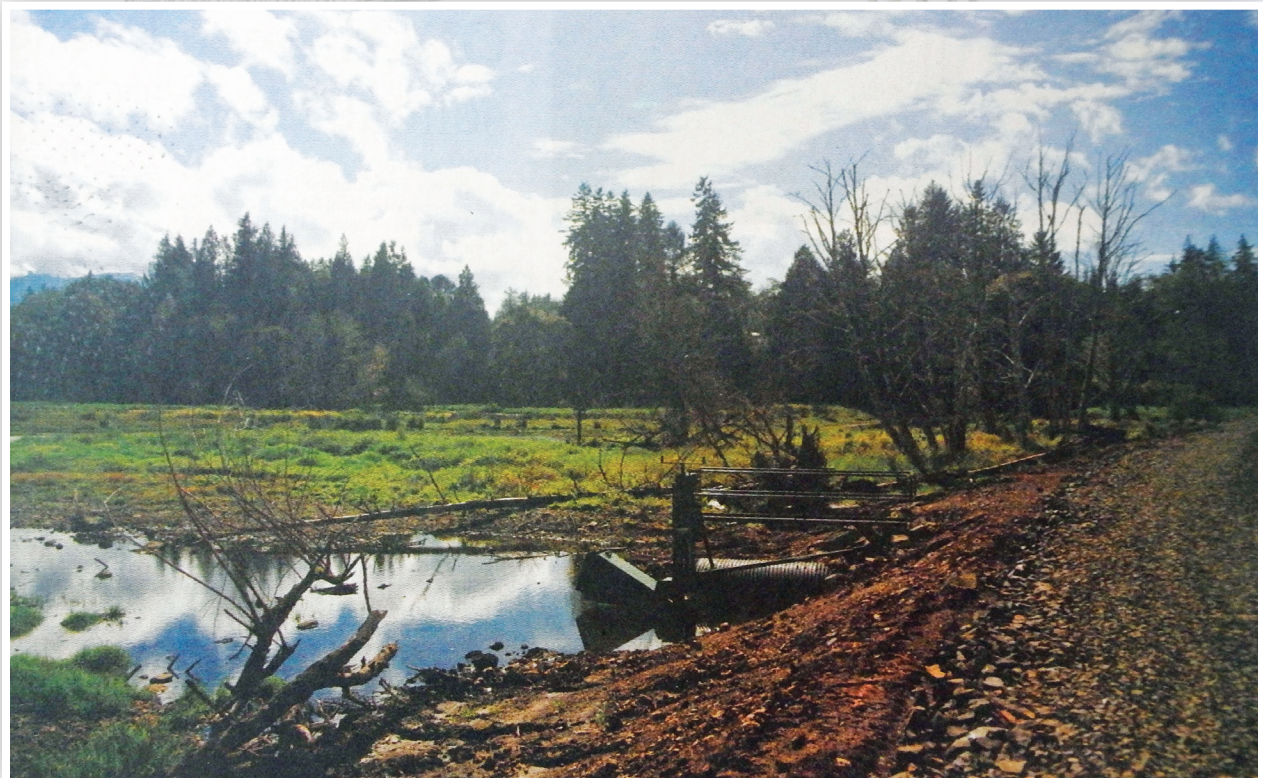
The newly installed tide gate at Warren Slough regulates water flow into Gary Ziak's field in Knappa in 2010.
