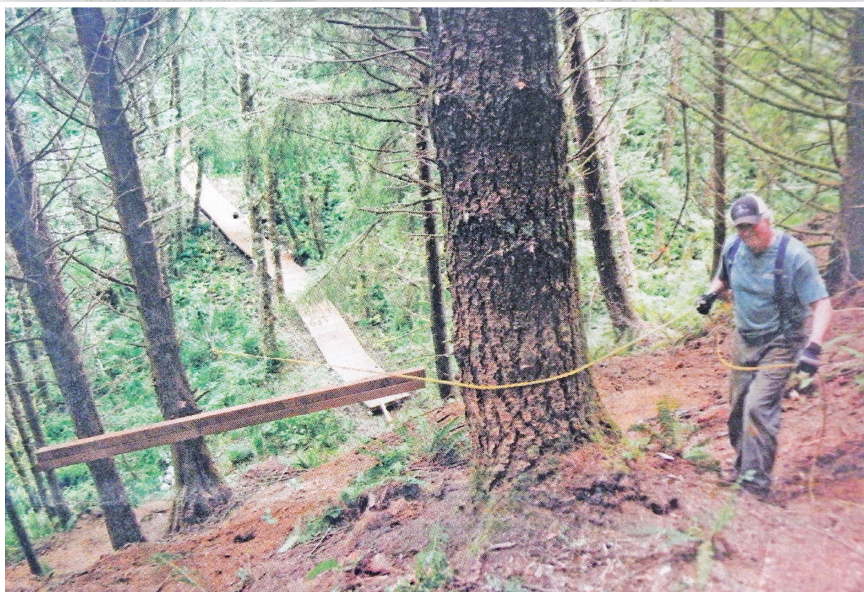
Dick Halverson lowers a pair of wooden beams down a steep hill using a cable zip line system during construction of a new trail at Lewis and Clark National Historical Park in 2010.
