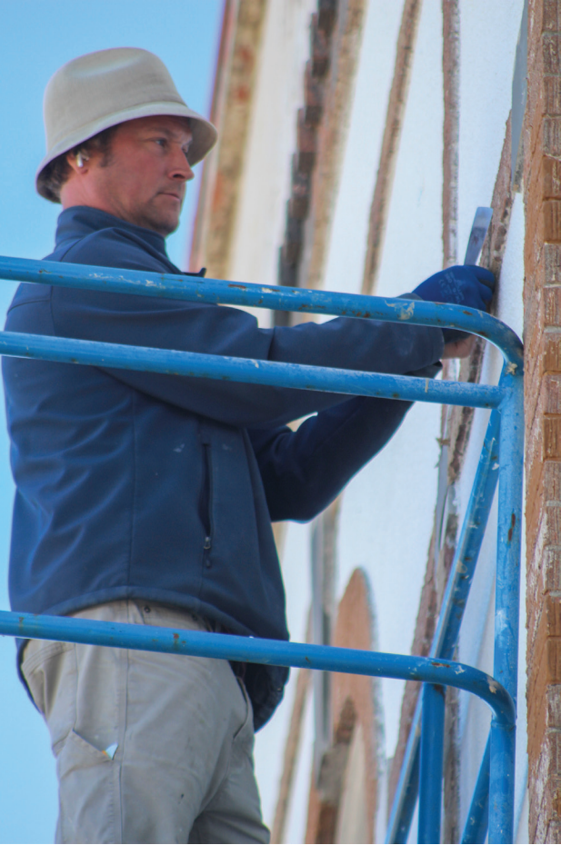
Edward Stratton/The Astorian The partners behind the restoration of the Odd Fellows Building in Astoria hired local contractor Simo Ranta to apply a new coat of paint.
