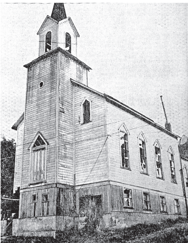
The Astoria City Council gave permission to demolish the old Zion Lutheran Church on 18th Street in 1970.
