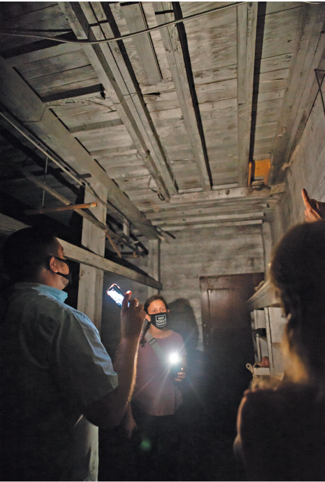
From left, Rainier Reyes, Nathalie Kellow and Diana Gulley inspect a trap door leading from the building above to the basement.
