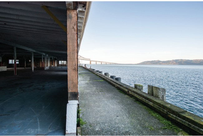
Hailey Hoffman/The Astorian Construction of the Bowline Hotel near Buoy Beer Co. is one of many construction projects happening in Astoria this year.
