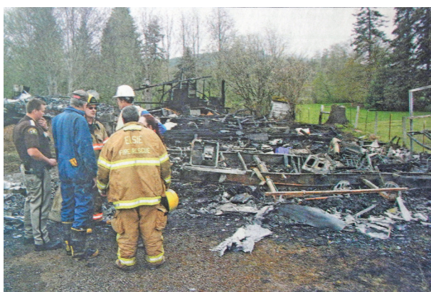
The Clatsop County Fire Investigation Team investigates a fire that started at 2:30 a.m. Saturday that destroyed the former Jewell Grange building.
