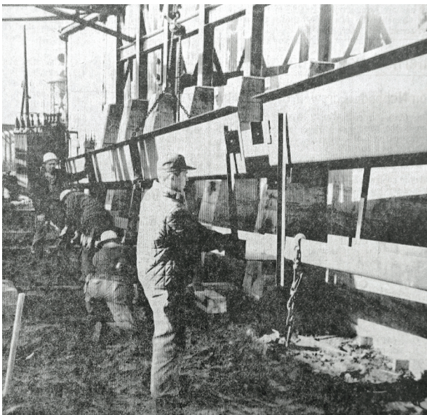
Workers move a conveyor into place on the Warrenton Lumber Co. construction project in 1970. From front to back are Ernest Mickle, Milford Mickie, Dude Hamilton and Si Jones.
