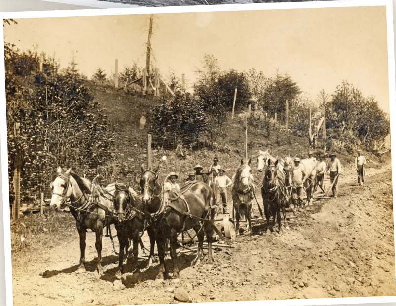
TOP LEFT: Altoona-Pillar Rock Road runs along the Columbia between Rosburg and the Pillar Rock Salmon Cannery. TOP RIGHT: Surveyors work on a wooden bridge somewhere between Knappton and Naselle, circa 1900. ABOVE: Norwegian immigrant Ole Dosland and his crew used horsepower to carve what would later become Washington state Route 4.
