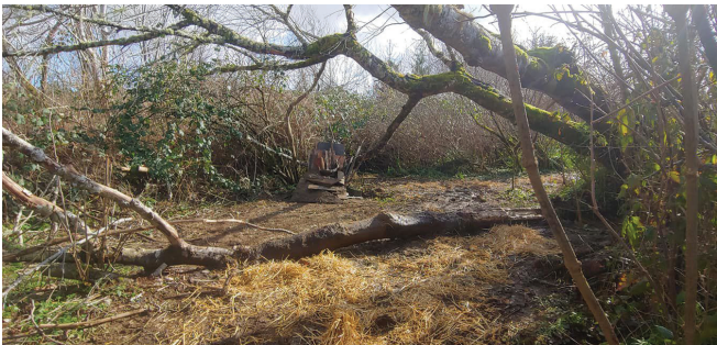
The cleanup at Mill Ponds after work by Jesse Anderson, Seaside Public Works and volunteers.
