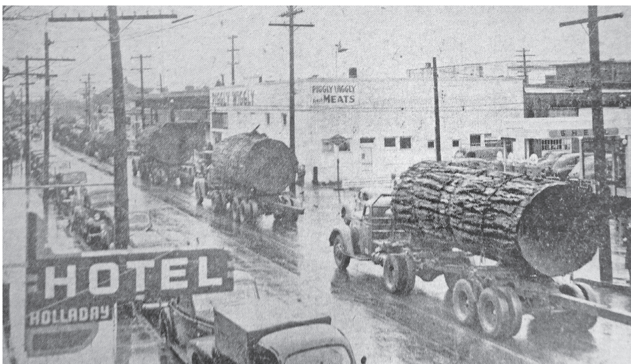
Part of the mile-long parade of 80 loaded log trucks trucked 400,000 feet of gigantic fir, spruce and hemlock sticks through Seaside during the Pacific Logging Congress.
