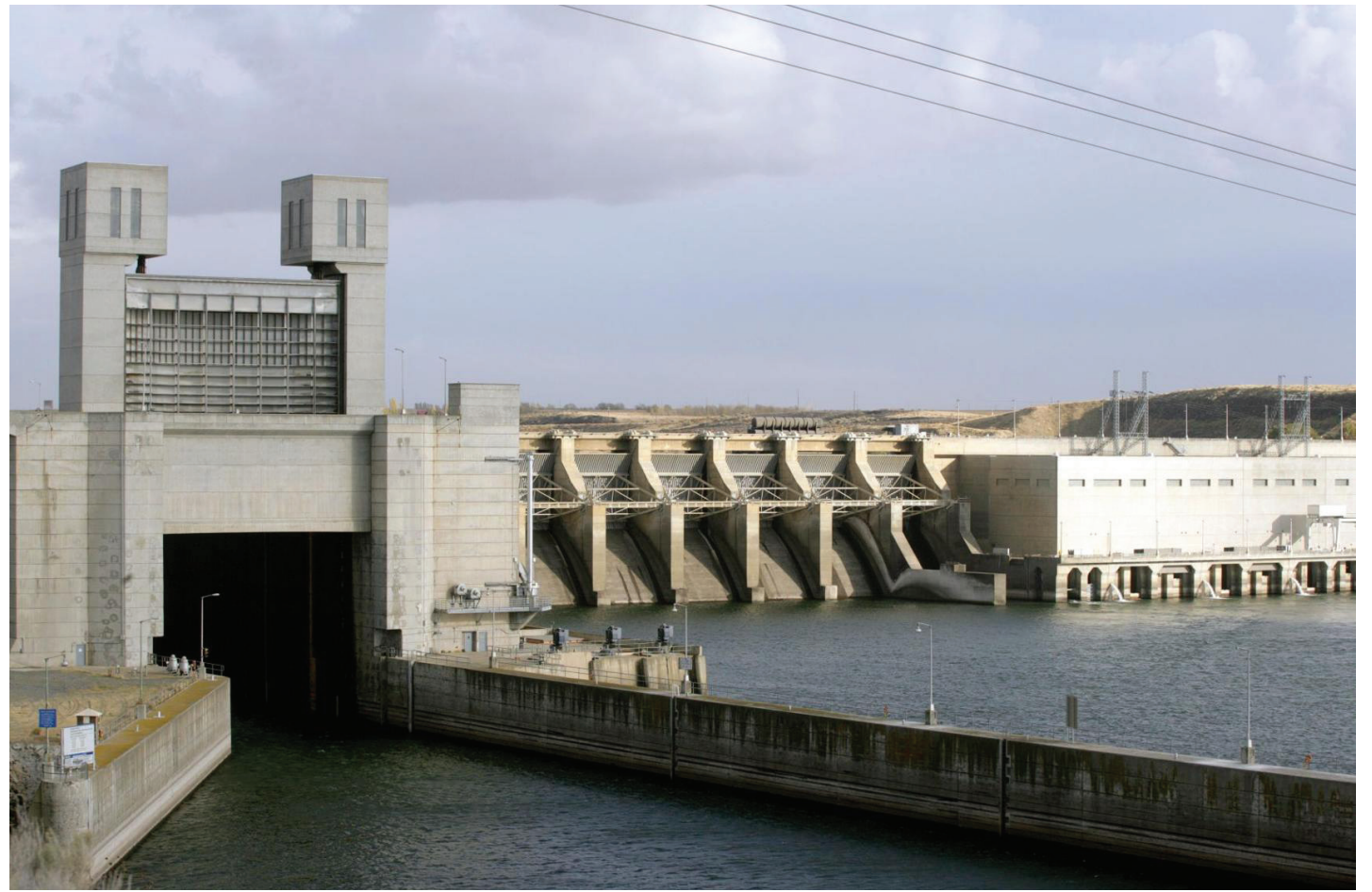
The Ice Harbor dam on the Snake River near Burbank.
