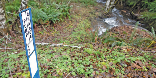
Astoria used federal emergency funds to repair erosion along Little Bear Creek threatening its main water transmission line.
