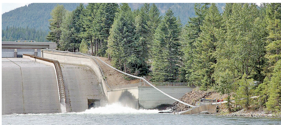
A tube carries fish over the Cle Elum Dam in July 2017. The 1,700-foot-long tube is the longest Whooshh Innovations has used to transport salmon. Fish travel at 32 feet per second.
