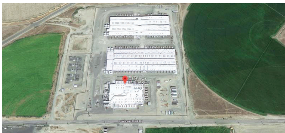
This Amazon data center site outside Boardman is one of seven operating or planned complexes in Eastern Oregon.
